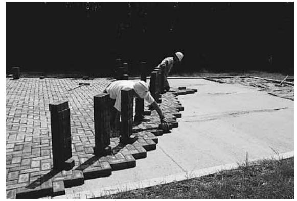
Figure 7. Placing the concrete pavers.
