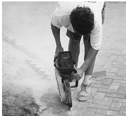
Figure 8. Saw cutting pavers.
