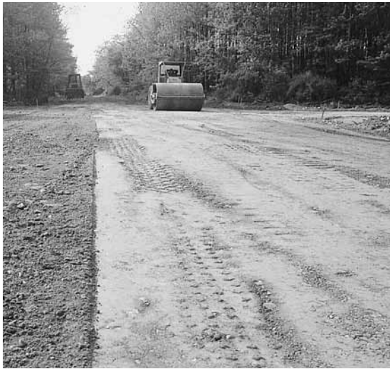
Figure 2. Compacting the soil subgrade.
