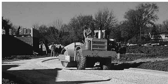
Figure 4. Base compaction with a vibratory roller.
