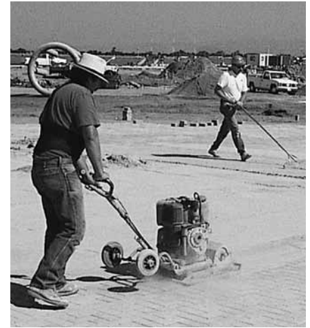
Figure 11. Vibrating sand into the joints.
