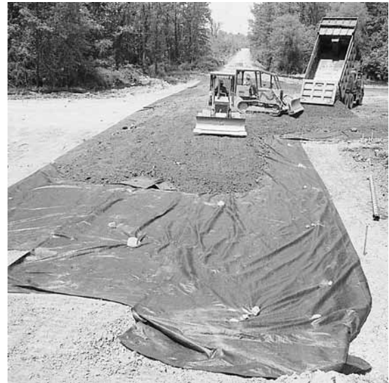
Figure 3. Application of the geotextile under aggregate base.
