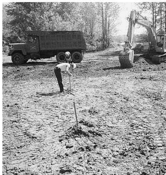
Figure 1. Excavation of the soil subgrade.
