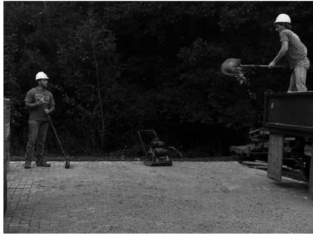
Figure 10. Spreading and sweeping joint sand.
