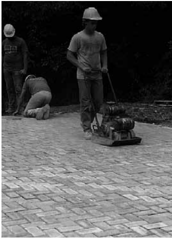
Figure 9. Compacting the pavers and bedding sand.
