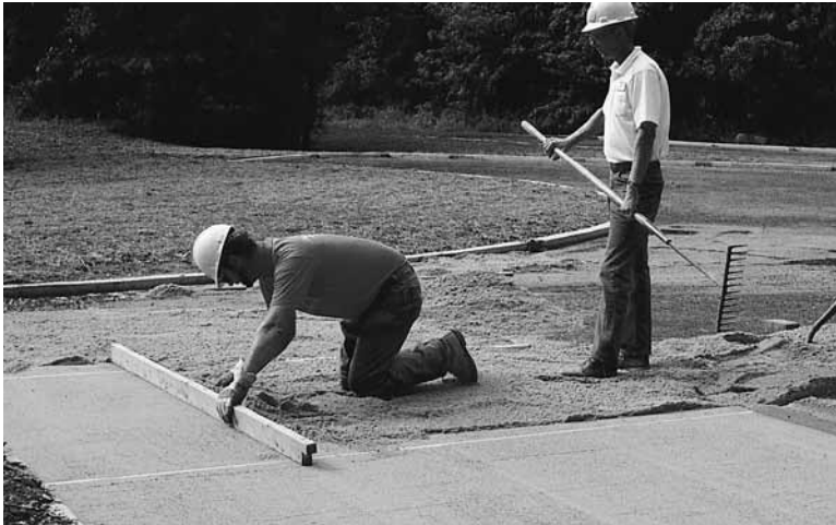
Figure 6. Screeding the bedding sand.
