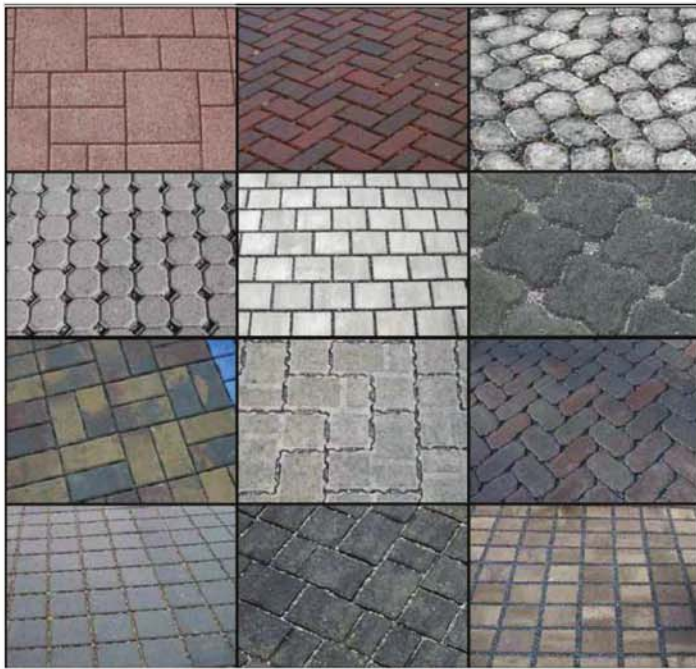
Aesthetic options abound for PICP installations, with little limitation in style, color, or shape.
